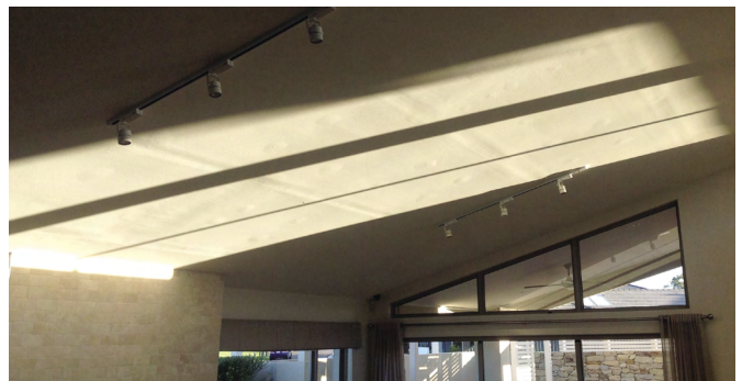
Figure 8: Same Plasterboard Surface Under Glancing Light
