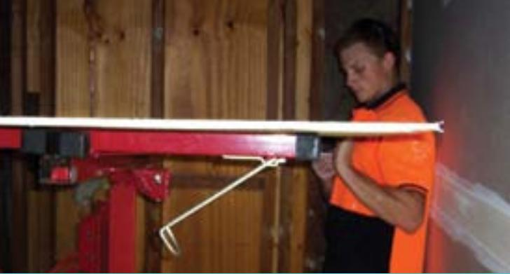
A sheet lifter is a simple and economical solution to the problem of placing and fixing ceiling plasterboard.
